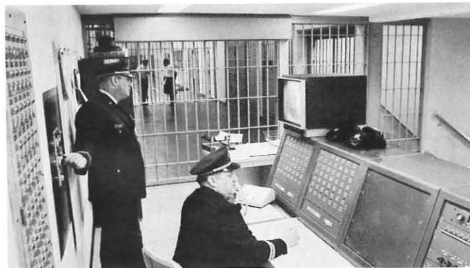
Security officer at the Baltimore City Jail's communications center confers with a guard via the prison's new Security Alarm System. All phones within the facility are linked to the communications network. Lights on the console indicate reports incoming from various stations, as well as telephones in use. The guard at left is handling controls for electrically operated doors. The closed circuit TV screen above the console provides a constant view of the entrance to the prison's maximum security section.
